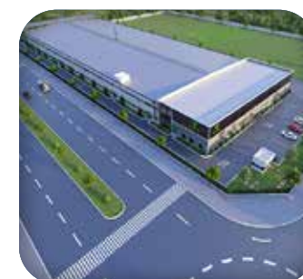
YAMAGATA Investor/main contractor: Yamagata Vietnam Co., Ltd Address: Yen Phong IP Bac Ninh
