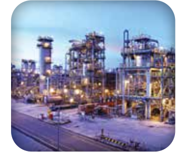
LONG SON PETROCHEMICAL Investor/main contractor: Long Son P.I.C Address: Ba Ria, Vung Tau
