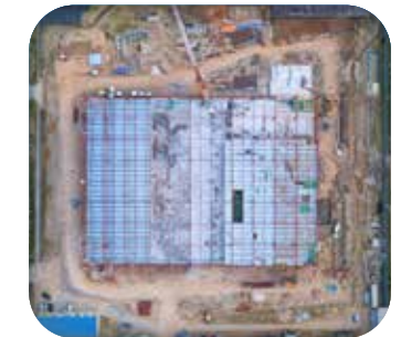
WELVISTA Investor/main contractor: Sungdo ENG Viet Nam Address: Bac Ninh
