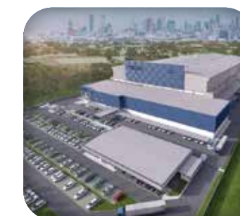
LTG Investor/main contractor: Thai Nishimatsu Construction Address: Samit Prakan Thailand
